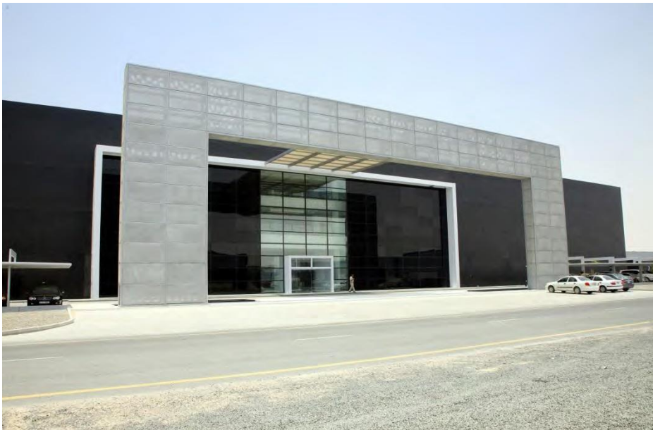
Warehouse Offices at JAFZA
