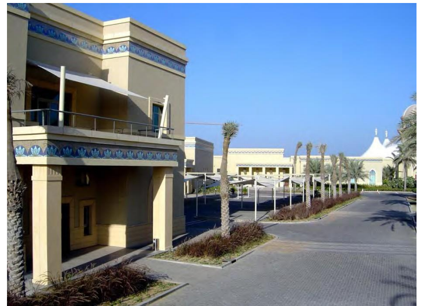
Nakheel Sales Centre Offices
